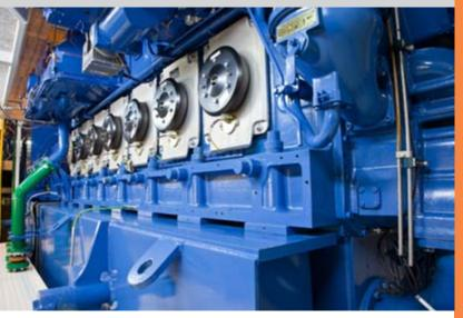
makes it possible to apply early inlet valve closure at high load, which in turn enables minimized NO<sub>X</sub> levels and reduced fuel consumption. By switching to late inlet valve closure, good part load and transient performance is assured. The overall operational benefits include improved part load performance, smoke reduction, and improved load acceptance.
