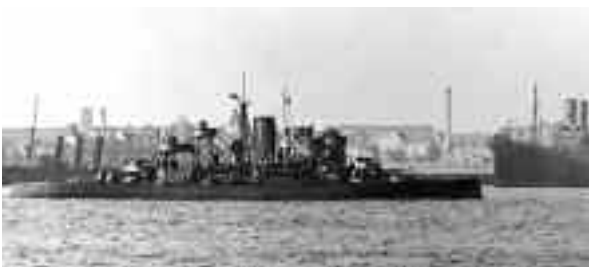
Thetis in the inner Kiel fjord in the autumn of 1942, painted in grey overall. Her forward searchlight appears to be covered by a tarpaulin, which renders it nearly invisible against the background. Hoods have been fitted to the directors, as well as splinter shields to the guns, and there is now a main topmast. Visible in the background are the hulked cruiser Berlin and the Hamburg-Amerika liner New York , both in use as accommodation ships. Shortly afterwards, Thetis would leave for northern Norway. (Dirk Nottelmann collection)
