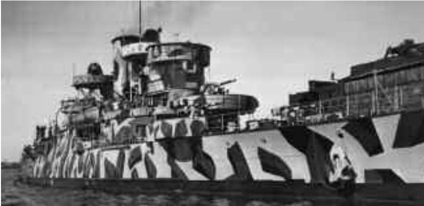
Thetis during the final stages of her fitting-out at Kiel. Her unique tripod mainmast has still to be erected. The photo gives an excellent view of the elaborate camouflage pattern with which she entered service. (Aidan Dodson collection)
