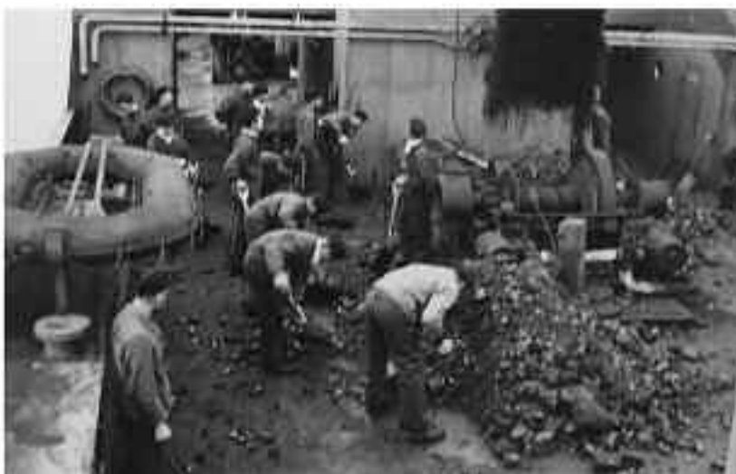
A set of images taken on board Medusa early in her career in 1940. Clockwise from top right: the forward starboard 10.5cm HA gun, still unshielded; coaling on the quarterdeck – note the steam-operated cargo winch, added during her conversion; one of the diesel generators in a former machinery space, with the switchboard overhead; the ship's cutter and the after end of the bridge structure. (Dirk Nottelmann collection)
