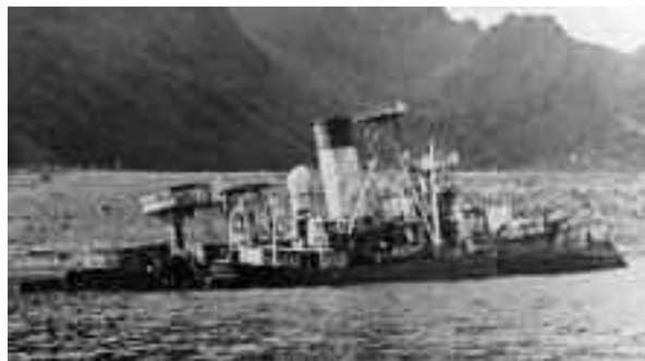
Nympe was run aground at Kunna, outside Svolvær, on 17 May 1945. She is shown here under salvage, with all significant fittings removed. An interesting detail is her heightened forward lattice structure, presumably intended to support a Würzburg antenna. Owing to her stripped state it cannot be verified whether this was ever fitted. (Aidan Dodson collection)
